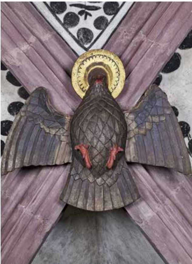
Fig.5: The central easternmost keystone: the Dove representing the holy spirit. Picture taken after cleaning and conservation. 2017, Nick Brändli.
