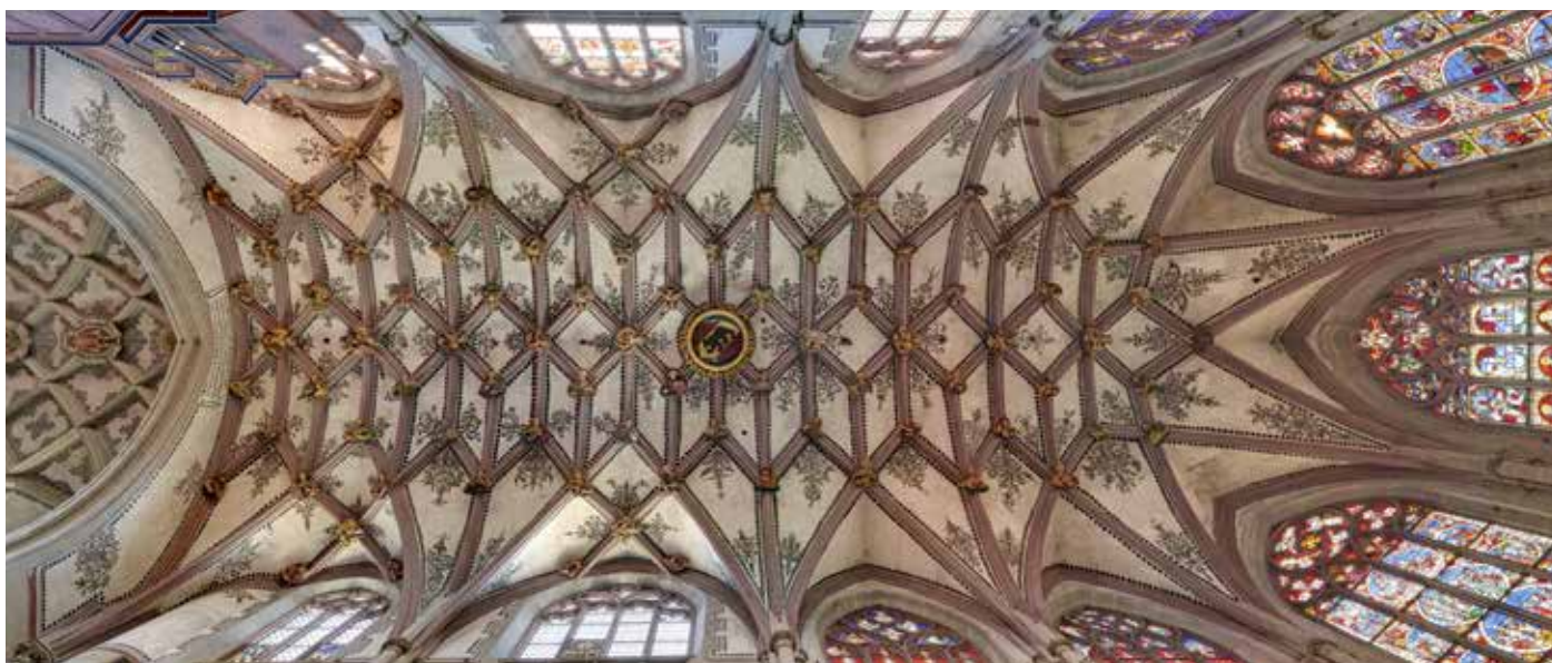
Fig.1: General view of the choir vault after conservation. 2017, Nick Brändli.
