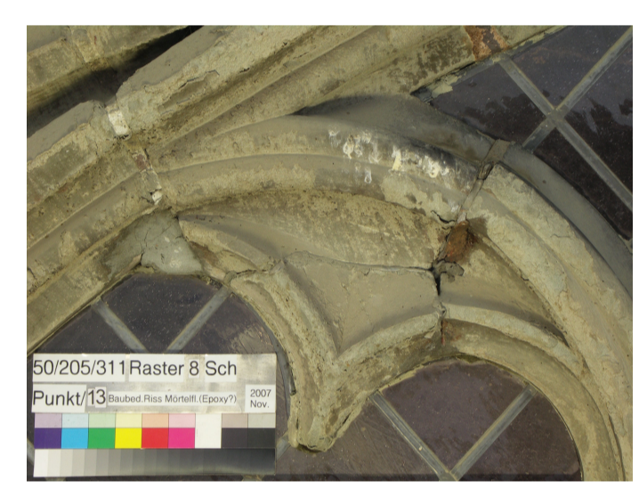
Detail 13: Alter Mörtelflick, Epoxid.
